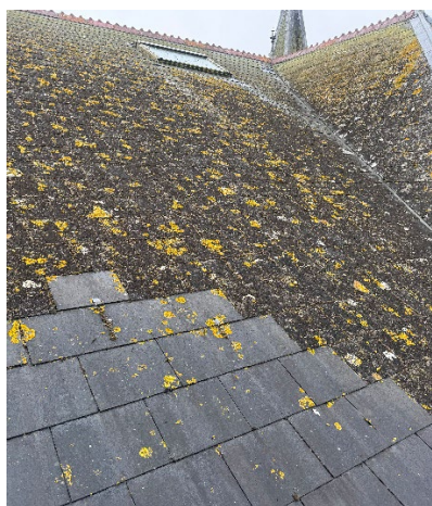
Fig. 3, Roof elevation photo 3
