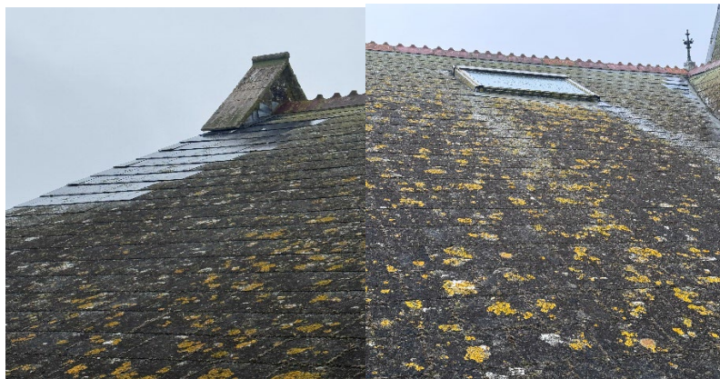
Fig. 1, Roof elevation photo 1 Fig. 2, Roof elevation photo 2
