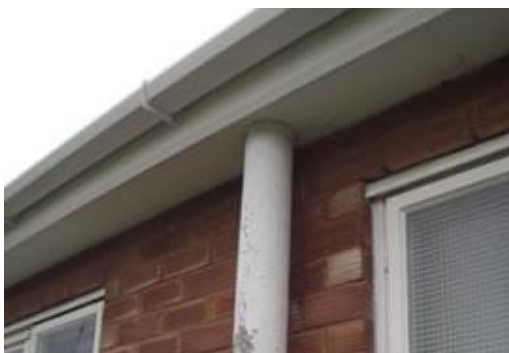
Asbestos cement drainage pipe (downpipe)
