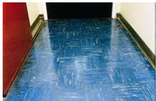
Asbestos containing floor tiles in a corridor
