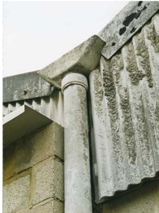
Asbestos cement downpipe, hopper and profile sheet
