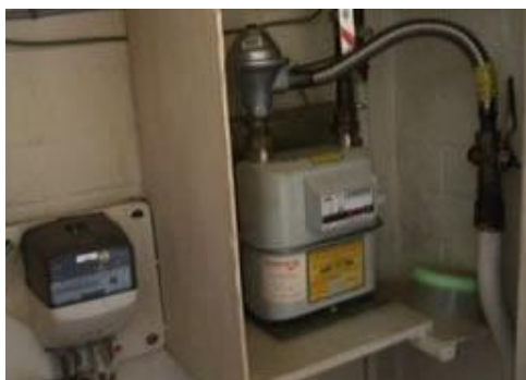
Asbestos panelling around a gas meter
