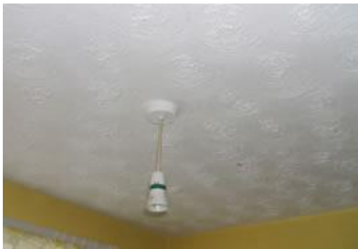
Asbestos textured coating
