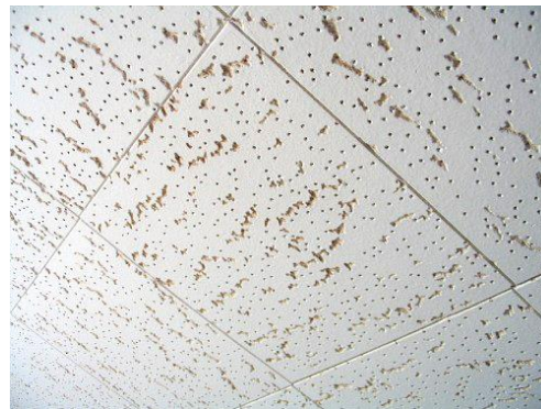
Asbestos containing ceiling tiles
