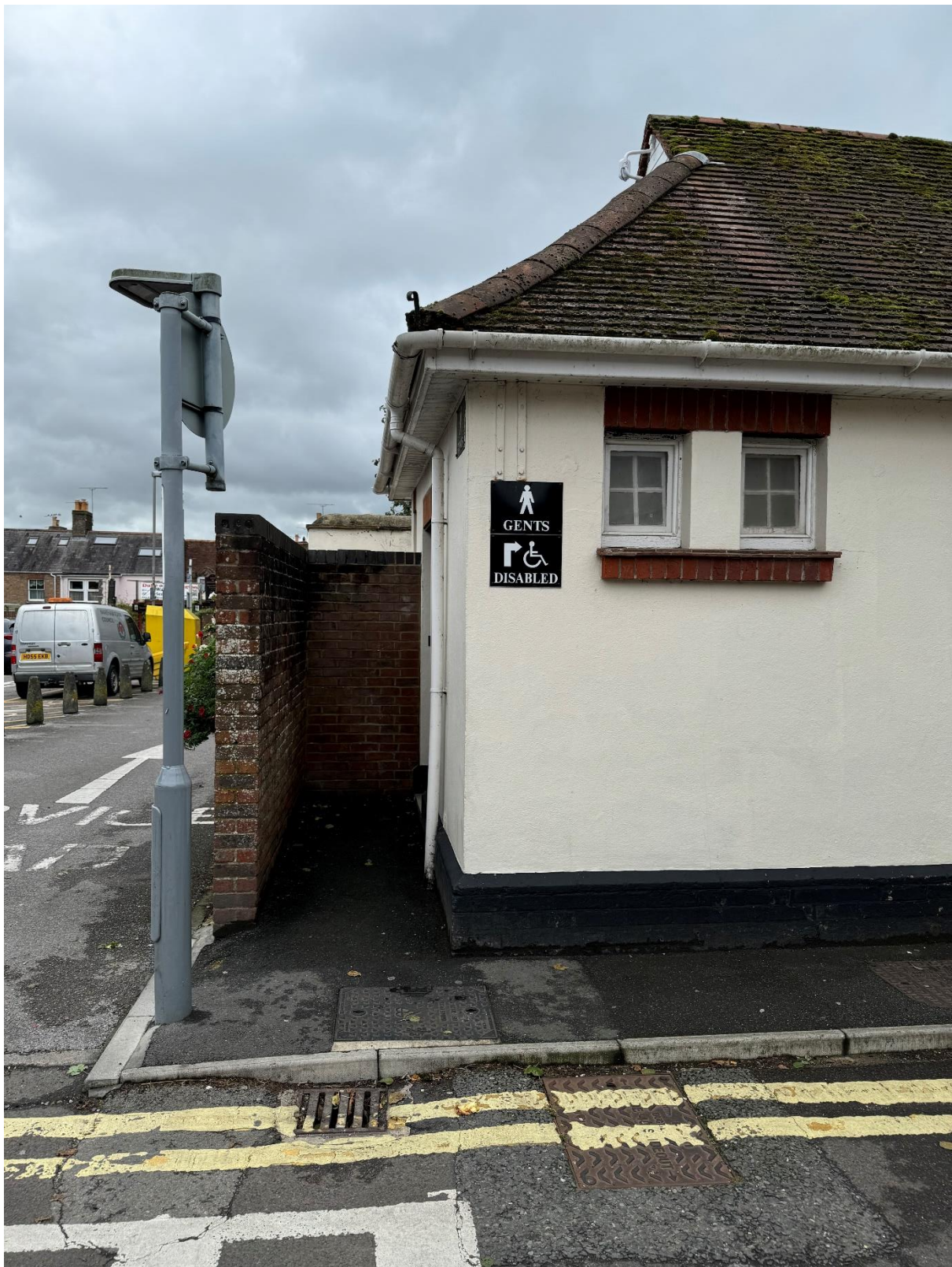
Front Profile Howard's Lane Toilets, Gents' Entrance nearest Howard's Lane Car Park
