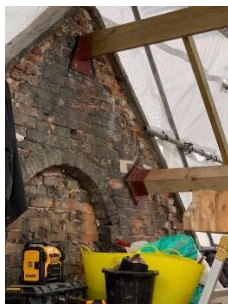
Photo 2 caption: Major structural beams and timberwork replaced before roof tiles replaced.
