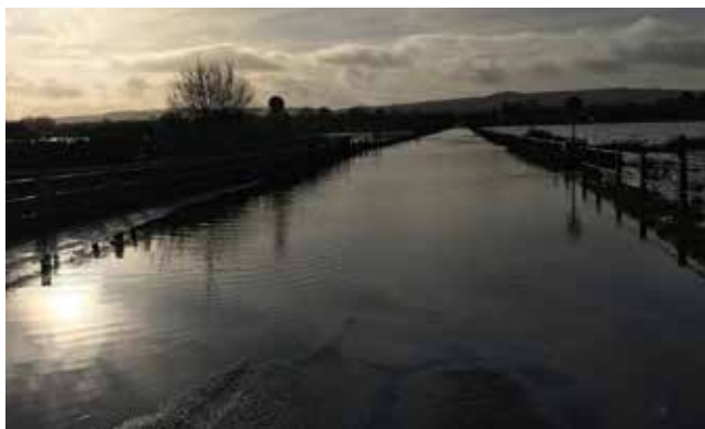
Figure 12: South Causeway Road Flooded January 2020
