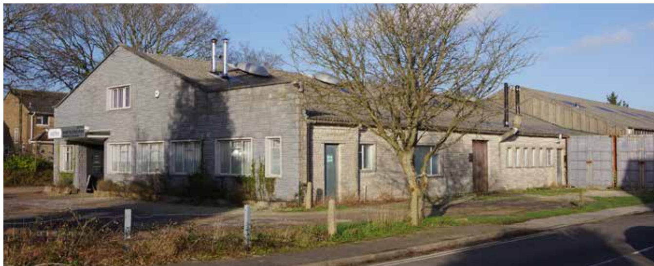
Figure 23: Johns Road Industrial Estate
